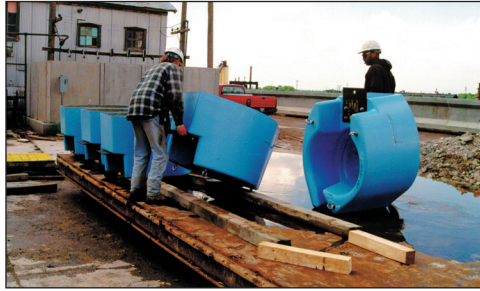
Step 2: Surface should protect lifting eye (sand, soft earth or blocks of wood)
