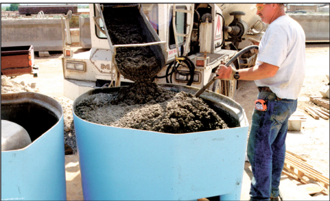
Step 4: Fill shell with concrete mix
