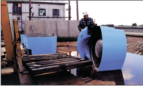
Step 1: Place fiberglass shell upside down on a prepared surface
