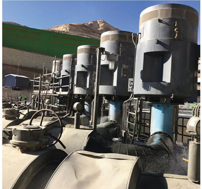
an average of 300 hours to over 1000 hours. The result was an increase in the MTBF of more than three times. The increase in overall pump life was largely driven by the Floway patented sealed-for-life bearing design, slurry mechanical seal, isolation device and hardened materials on the wear parts. In addition, the VTSP design eliminated the need for any type of external flushing, which prevented the risk of dry running the bearings and seals.
